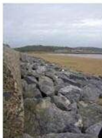
Rip Rap (Rock Armour)
