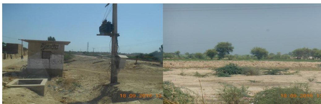
Railway Track at Project Area
