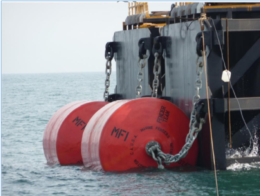
Figure 3.16: Breasting dolphin with foam filled floating fenders ©Shibata Fender Team
