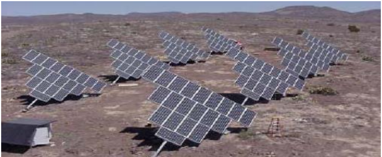
Figure 15 The polar axis tracker
