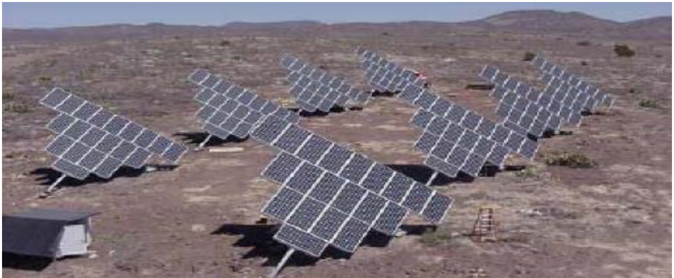
Figure 15 The polar axis tracker
