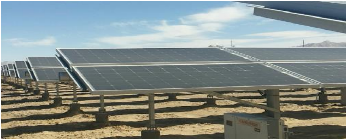
Figure 14 The horizontal single axis tracker
